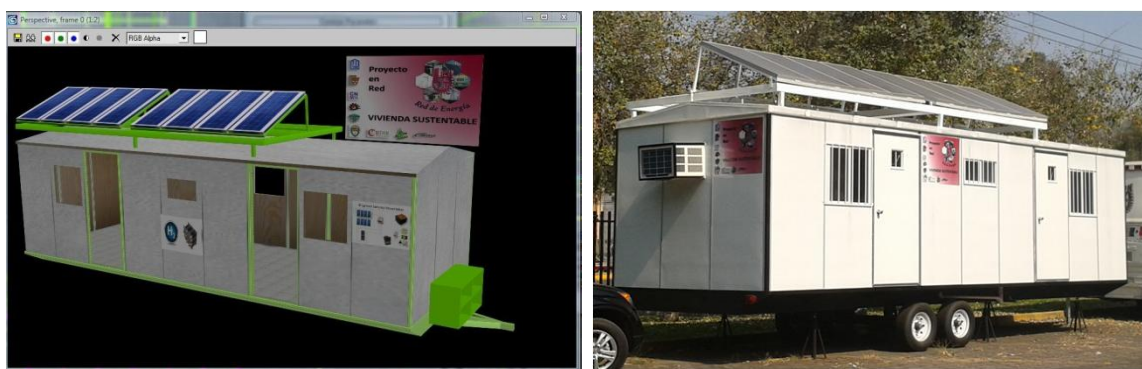
Figure 3. Sustainable house developed at IPN with a 1 kW solar photovoltaic system powering the house. Solar panels installed in the roof are made of polycrystalline Si.
